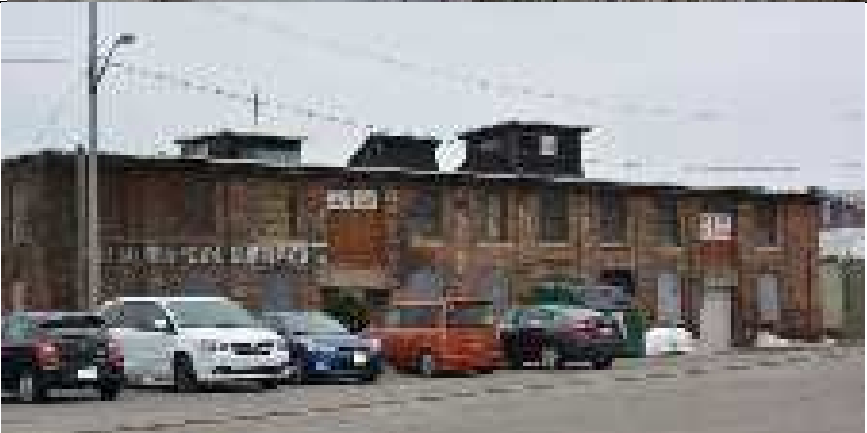
418 Lafayette Street, facing southwest
