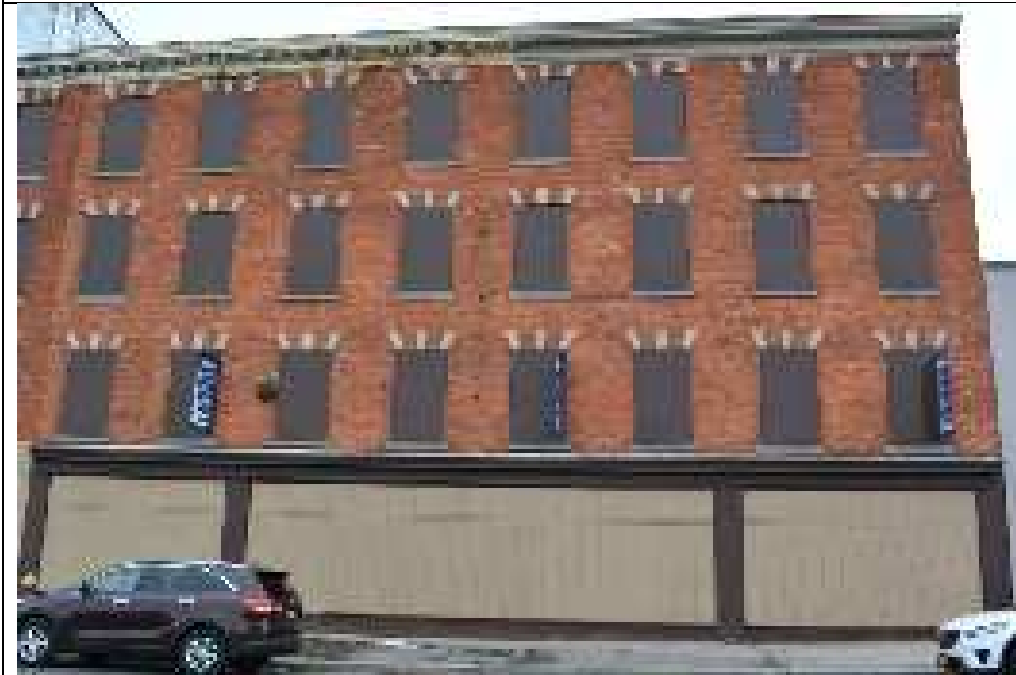
333 Lafayette Street, facing east
