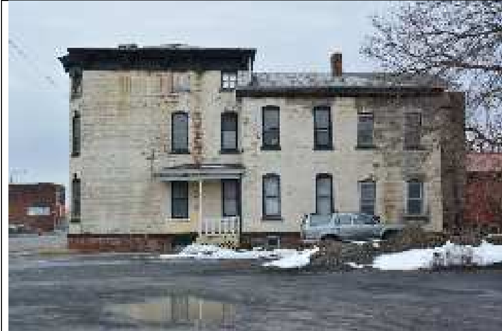
437 Lafayette Street, facing east
