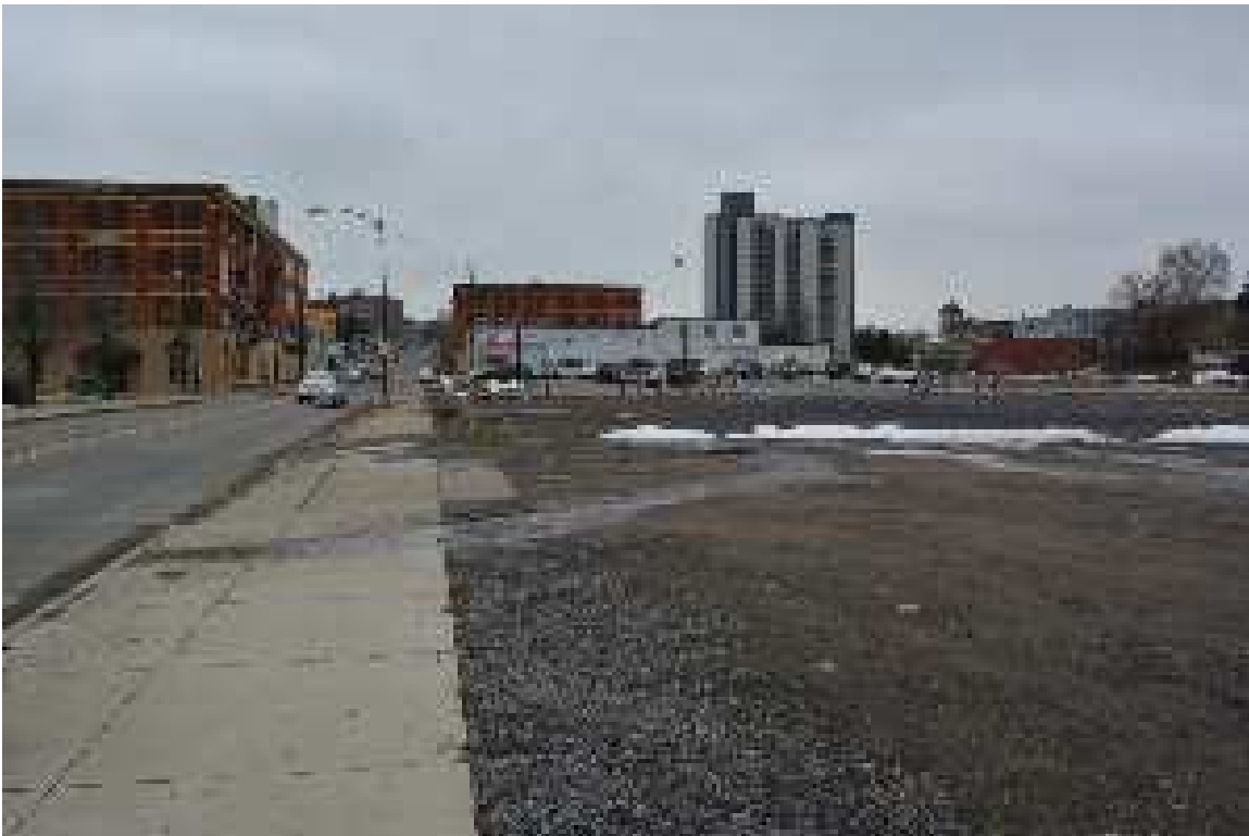
Photograph 8. Along Cornelia Street from Oriskany Street West, facing south (Panamerican 2018).
