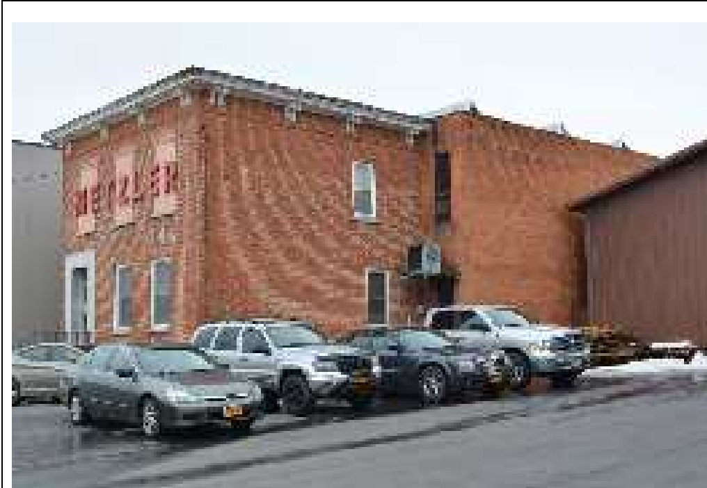
317 Lafayette Street, facing southeast
