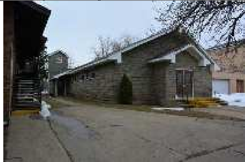
425-429 Lafayette Street, facing southwest
