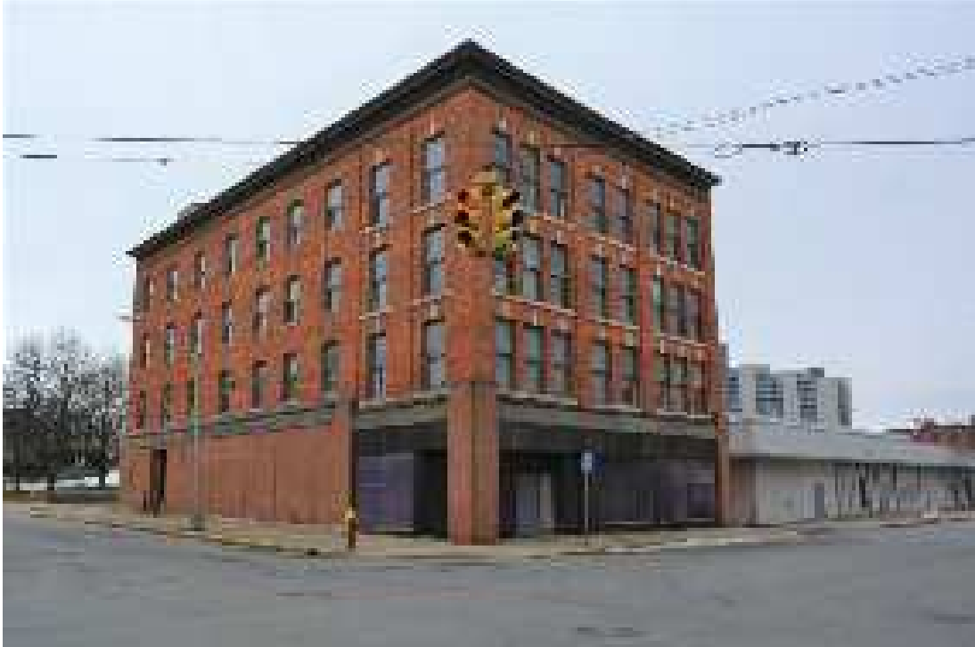
Photograph 3.3. Contributing building at 301 Columbia Street (USN 06540.002010) to the NRL Downtown Genesee Street Historic District, facing southwest ( Panamerican 2018 ).
