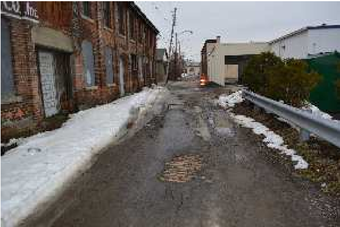
Photograph 16. View from east end of Carton Avenue, facing west. Note, exposed sandstone pavers in foreground (Panamerican 2018).
