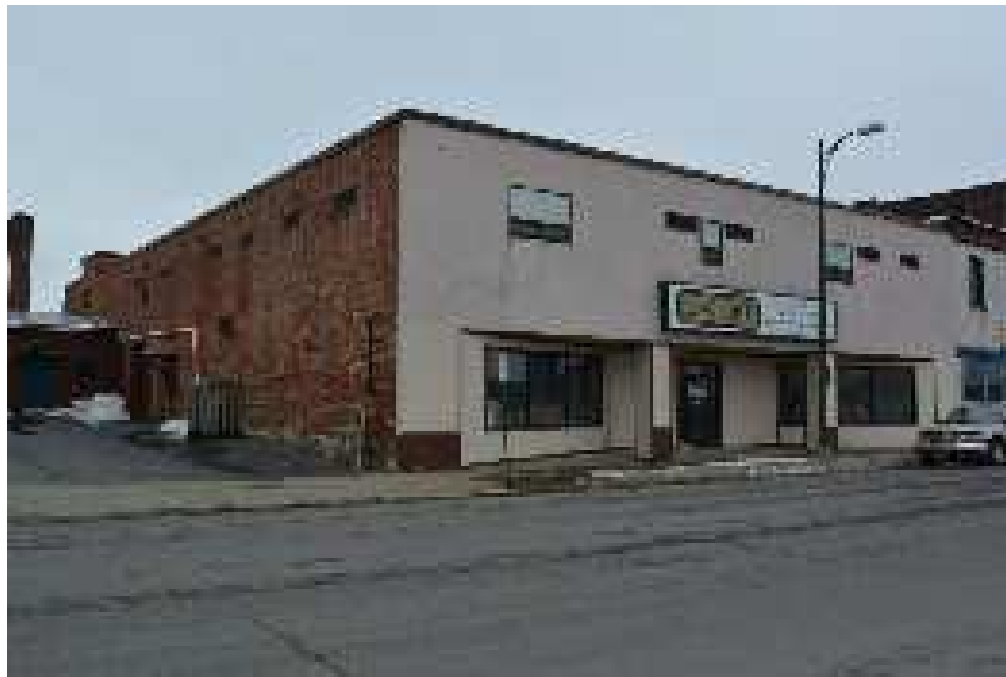
319-325 Lafayette Street, facing southwest
