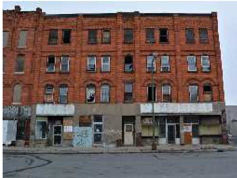
326-334 Columbia Street, facing north
