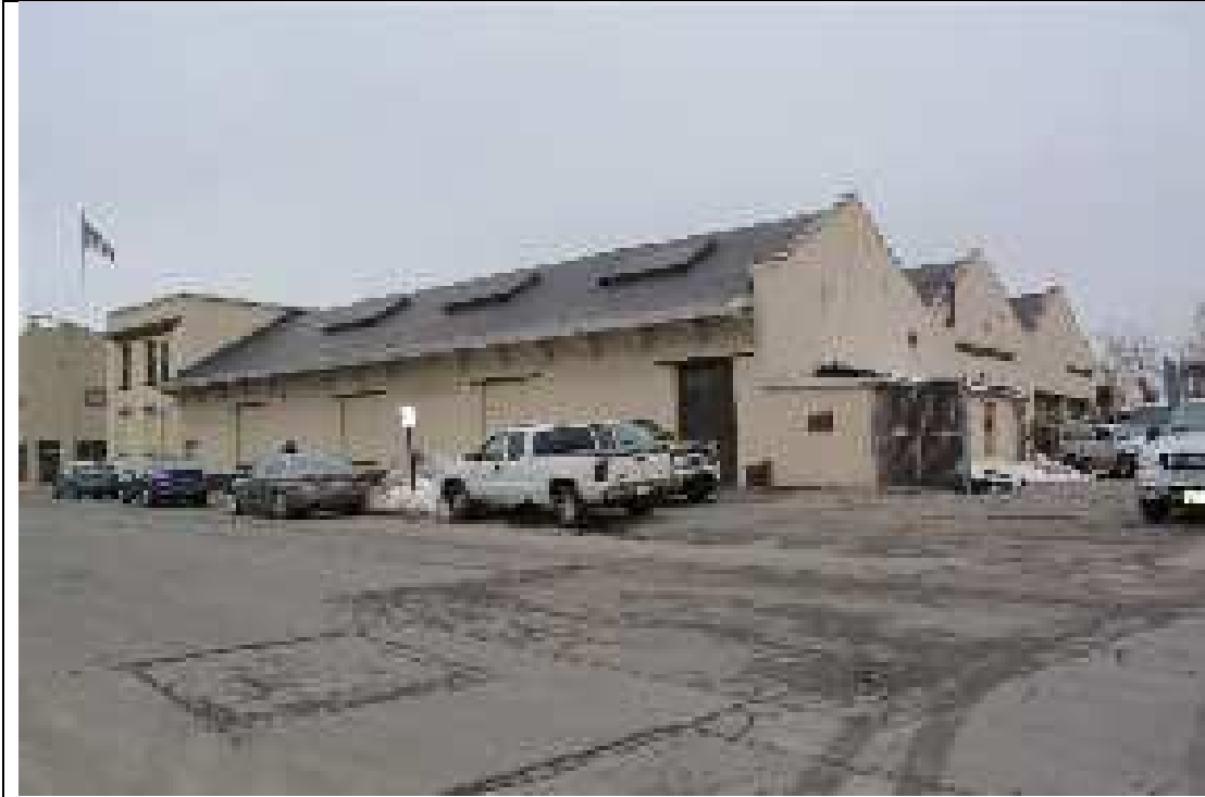
300-306 Lafayette Street, facing southwest
