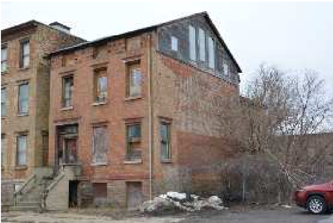
Photograph 3.7. L. Snyder House (ca. 1835) at 440 Lafayette Street, facing northwest (Panamerican 2018).
