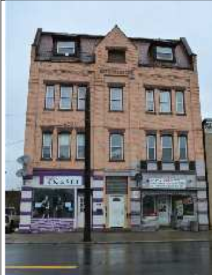
460-464 Columbia Street, facing north
