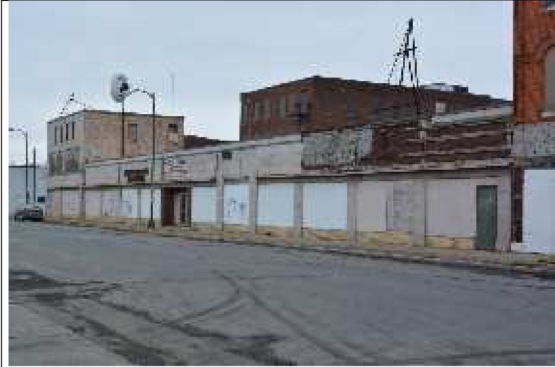
338-358 Columbia Street, facing northwest
