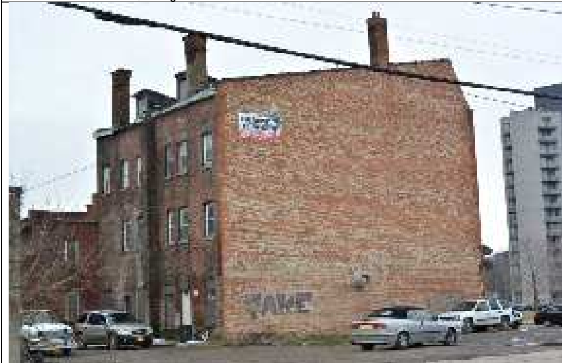
460-464 Columbia Street, facing southeast
