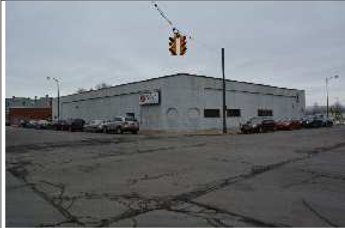
406 Columbia Street, facing northwest
