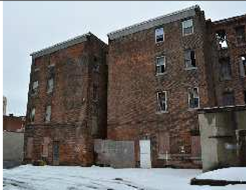
326-334 Columbia Street, facing southeast
