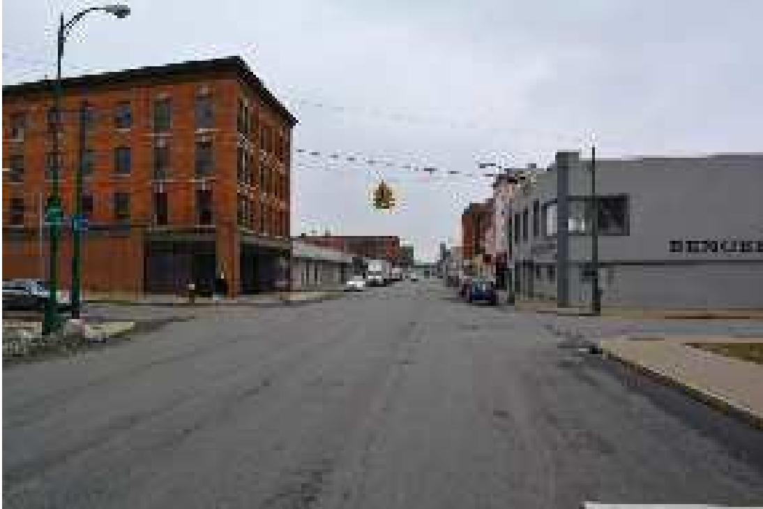
Photograph 3.1. View along Columbia Street from east of Broadway showing the section of the Downtown Genesee Street Historic District between Broadway and Cornelia Street, facing west ( Panamerican 2018 ).
