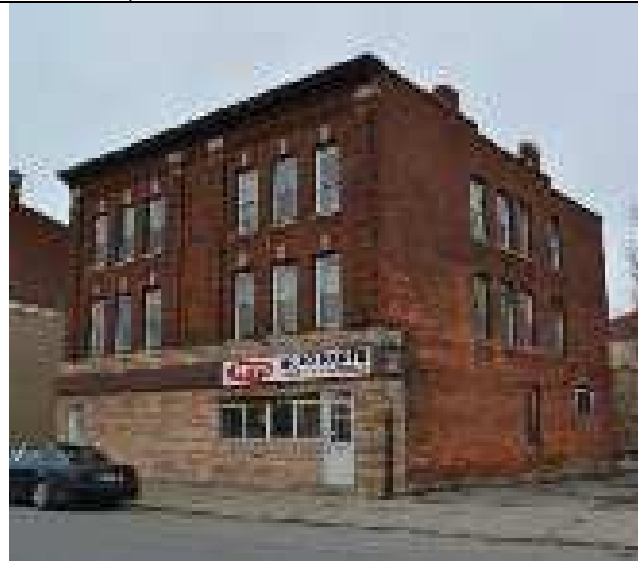
452-454 Columbia Street, facing northwest
