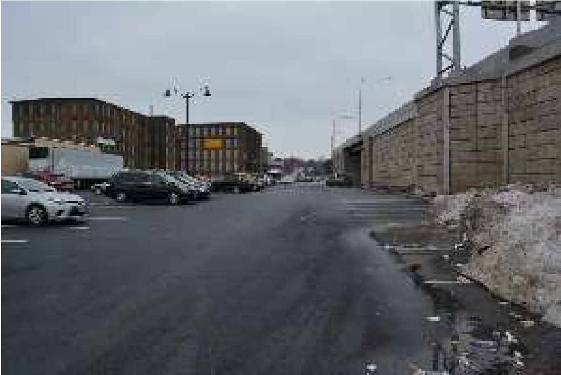
Photograph 23. Northwest limits of Project along State Route Highway 5 overpass, approximate location of former Chenango Canal, facing south from Lafayette Street (Panamerican 2018).
