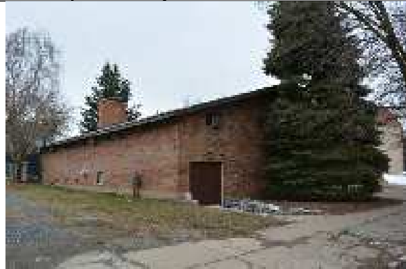
425-429 Lafayette Street, facing southwest
