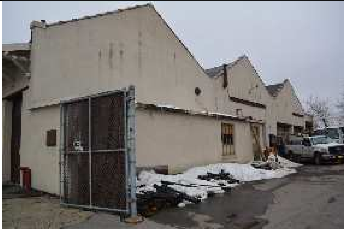
300-306 Lafayette Street, north side, facing southwest
