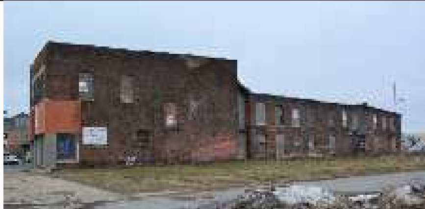
418 Lafayette Street, facing west-northwest
