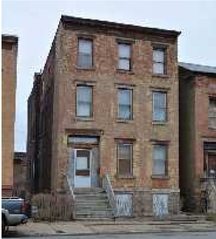
Photograph 3.8. Isele House (ca. 1835) at 442 Lafayette Street, facing north (Panamerican 2018).
