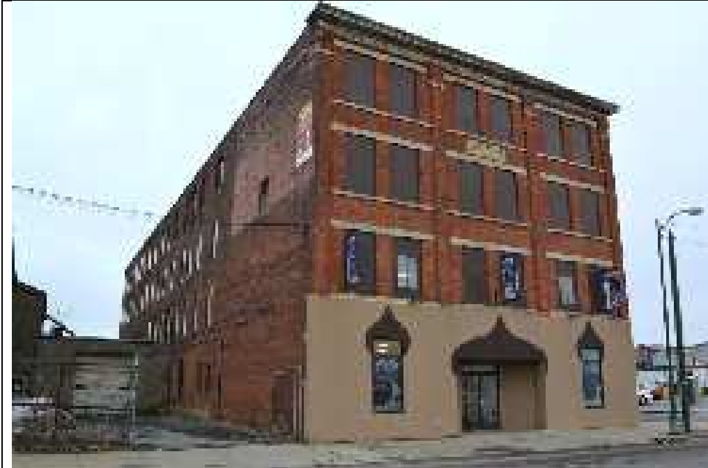
333 Lafayette Street, facing southwest
