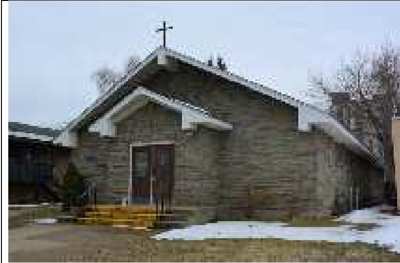
425-429 Lafayette Street, facing southeast
